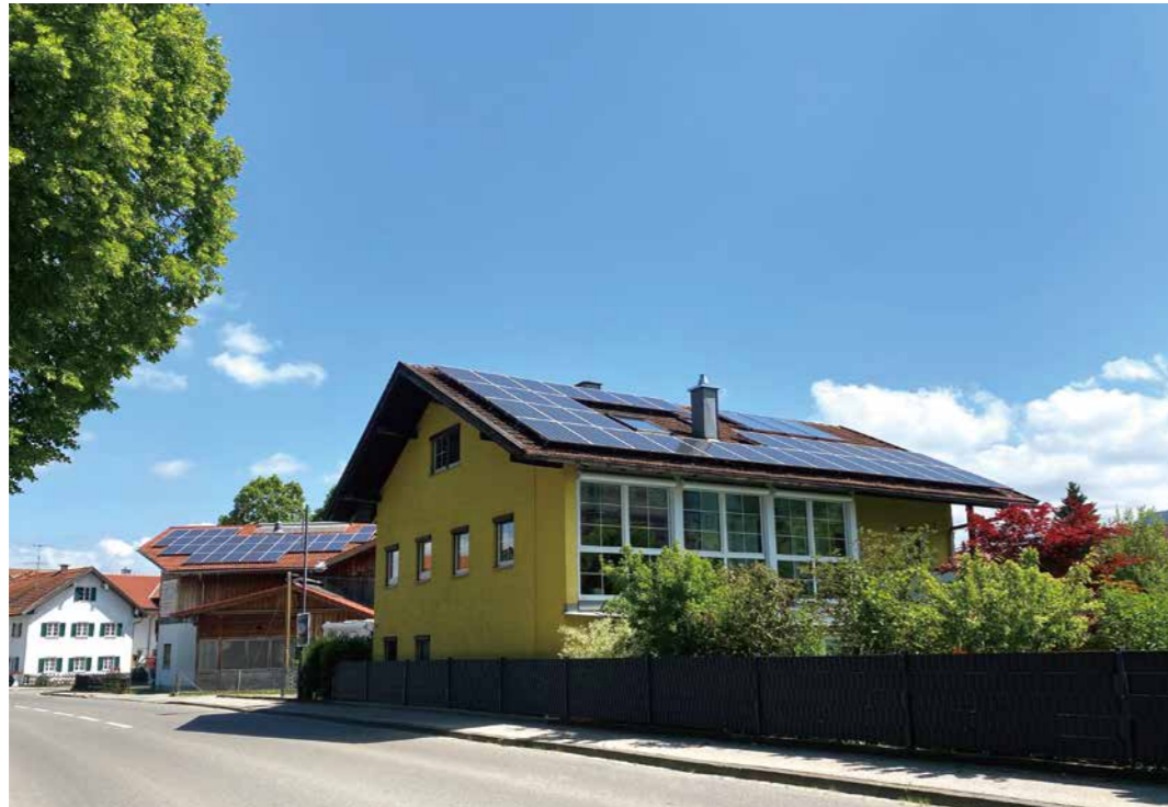
08 Residential ESS Project in Europe
