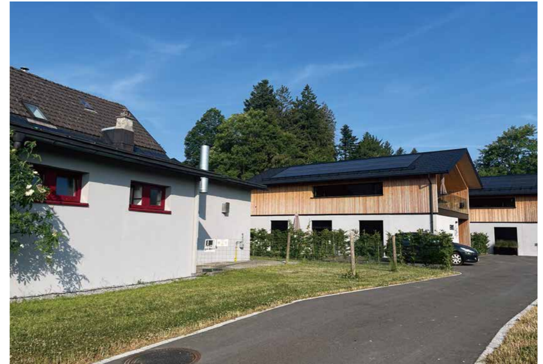
09 Residential ESS Project in Europe
